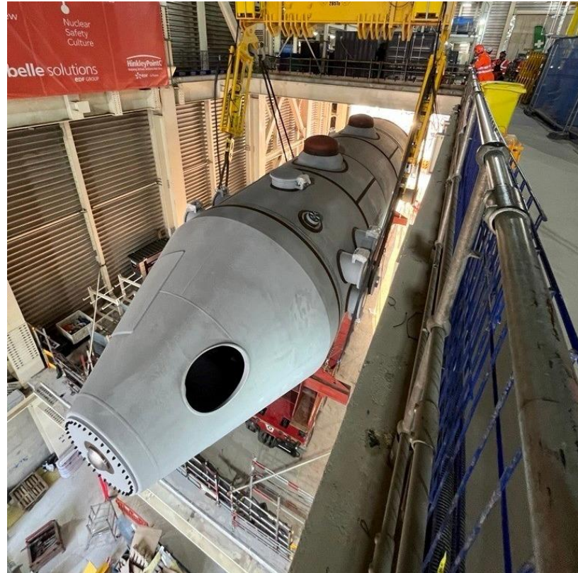
The 22-metre high MSRs were manoeuvred into place using the turbine hall's 300-tonne gantry crane.
