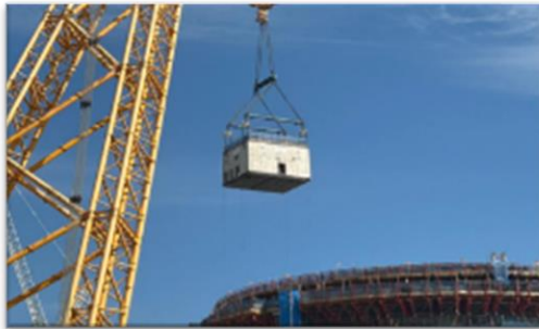
Above: Modularisation now includes whole pre-cast rooms,
